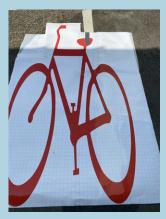
The bike sharrow installation template allows the one team member to align the pre-formed thermoplastic bike sharrow symbols on the printout while another crewmember preps the pavement, and then slides it right into place. The new process requires very minor adjustments and takes about half the time of traditional placement.
