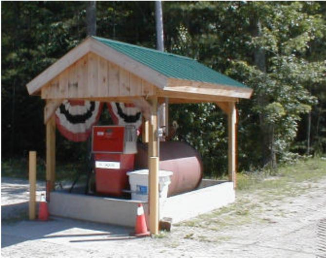
*A fueling station at a typical NH Highway garage. A cover over the fueling area is needed to comply fully with NHPDES II.*
