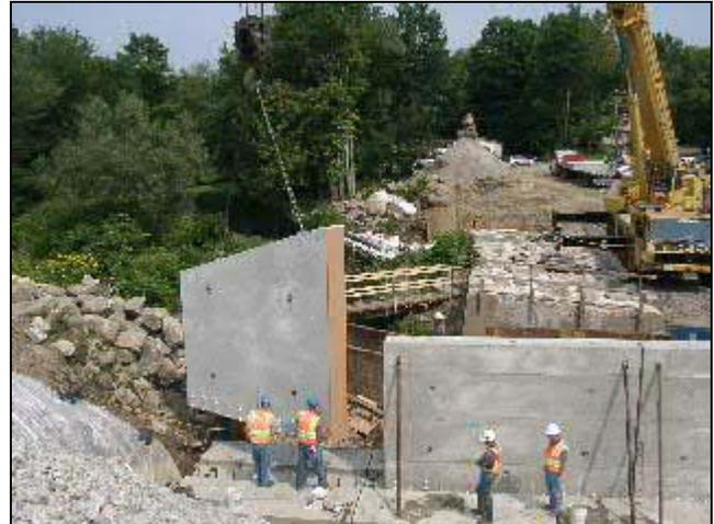
Each abutment and wing wall section took three quarters of an hour to grout.
