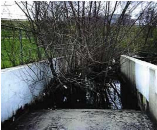
**Trees growing out of this concrete influent channel leading into a large extended detention basin in Austin, TX, indicate that maintenance has not been performed regularly at this site. In addition, the design of the channel allows a permanent pool of standing water to form behind the concrete riser. The combination of stagnant water and vegetation is highly attractive to mosquitoes.**
