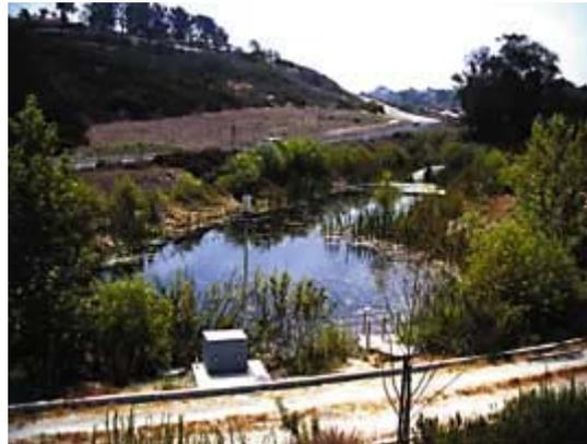
**Emergent vegetation such as cattails can rapidly overrun and clog retention ponds and constructed wetlands less than 4 ft. deep. This Caltrans site in San Diego County requires annual clearing of cattails that fill all but the deepest sections of the pond. This maintenance is necessary to reduce vector production and maintain the function of the BMP.**
