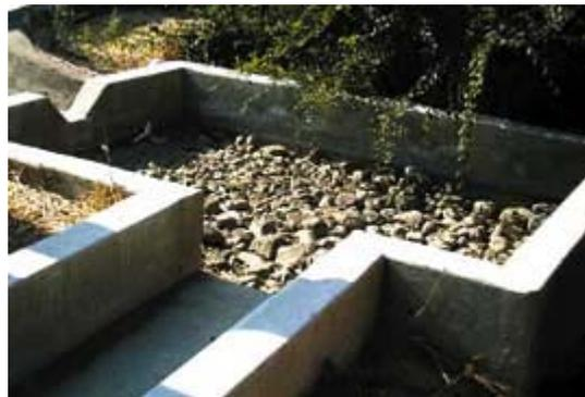
**The design of certain Caltrans biofiltration swales included concrete depressions used to house rocks for energy dissipation. These depressions held standing water for weeks and provided suitable habitat for hundreds of mosquito larvae. A workable solution entailed filling the depressions with concrete and embedding the rocks into it. This provided the necessary energy dissipation while eliminating the mosquito habitat. No mosquitoes have been detected at these sites since October 1999.**
