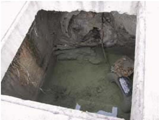
**Poorly designed underground stormwater junction where hundreds of mosquito larvae were found after a large storm**
