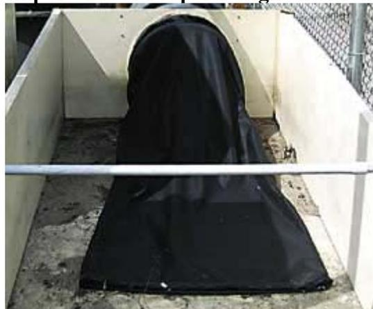
**CDS devices have a permanent water sump where trash and debris are separated from incoming stormwater runoff. This belowground habitat was attractive to certain species of mosquitoes and provided suitable habitat for thousands of mosquito larvae. Mosquito-proofing efforts were undertaken that included sealing off all entry points to the sump by using foam seals on lids and fine-mesh nets on the effluent pipe. No mosquitoes have been detected since January 2001.**
