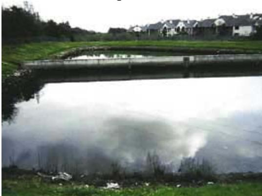
**Devices designed to completely dewater are prone to clogging over time if not regularly maintained. This giant Austin-type sand media filter in Austin, TX, was completely clogged. The resulting shallow lake was rich in organic debris and free of predators, providing a perfect mosquito and midge habitat capable of supporting millions of larvae.**
