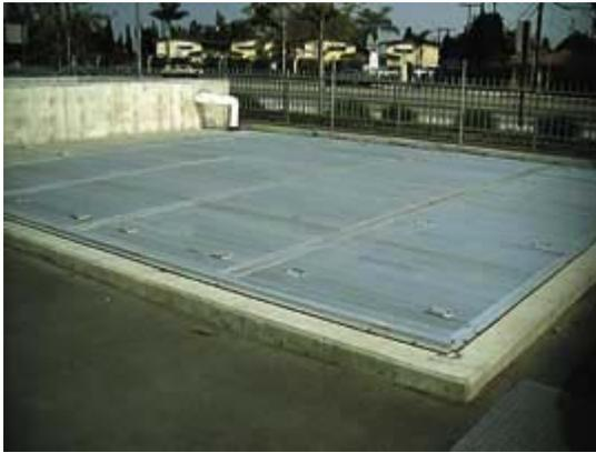
**The multichambered design of MCTT media filter devices prevented all but the last few feet of water to be pumped from the sedimentation chamber to the sand media chamber. The remaining water stagnated for months and provided habitat for tens of thousands of mosquito larvae. The retrofitted cover has been successful in excluding mosquitoes since March 2001.**
