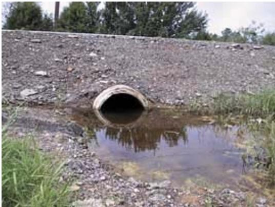
**Poorly designed culvert and eroded area with standing water likely to produce large amounts of mosquitoes**
