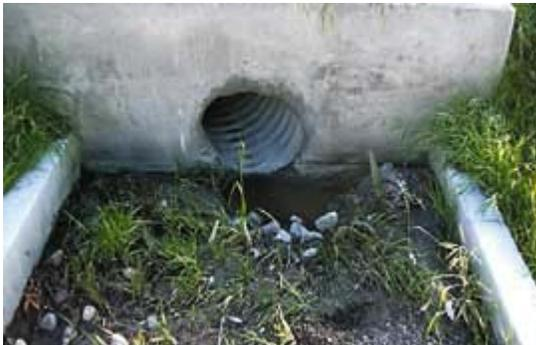
**Deposition of silt and debris can result in pools of standing water over time. This is the influent pipe leading from a major freeway interchange into a Caltrans biofiltration swale in Los Angeles County. This debris accumulated over the course of one year.**
