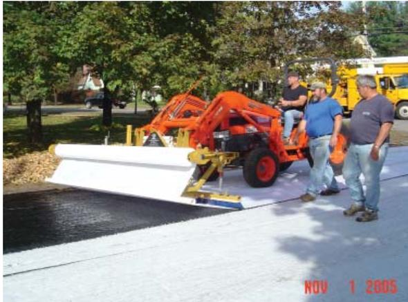
Good drainage is crucial to a road's performance. Water softens the subgrade and reduces its structural capacity. To control water infiltration into the subbase, agencies often use subsurface drainage and ditches or pavement seals. Although an overlay seals the pavement, overtime, reflective cracks will reappear. This article discusses the use of paving fabrics.
