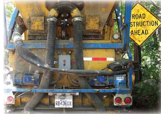
Back of the truck used on the FDR Project.
