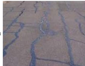
Decide whether a crack is “working” or “non-working” first in order to know whether to crack seal or crack fill. A “working crack” is a crack that has a large amount of horizontal movement. A “non-working” crack has a small amount of horizontal movement. Road managers should crack seal working cracks and crack fill non-working cracks.
