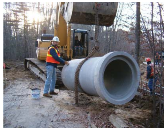
Culvert Installation
