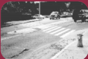
Pedestrian access is allowed only across the legs of the roundabout, behind the yield line.
