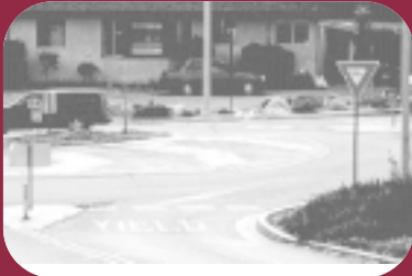
Yield control is used on all entries. The circulatory roadway has no control.
