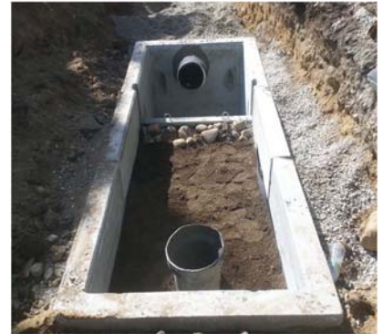
Media Box Filter with geotextile and pipe installation
