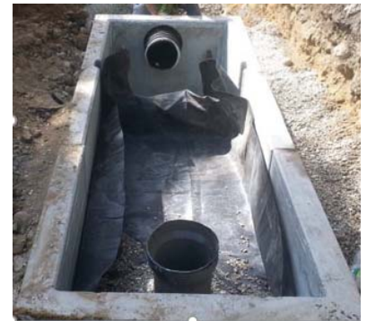
Media Box Filter with geotextile and pipe installation
