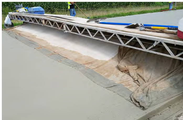
Fiber-reinforced concrete overlay with 4 lb/yd 3 of synthetic macrofiber and 4-in depth showing excellent finishability. Source: Iowa Concrete Paving Association (ICPA)
