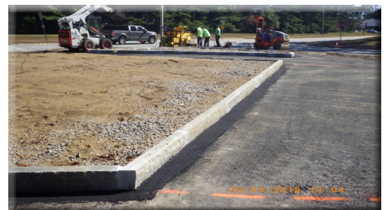
Curb installation and Paving, Fall 2018 Photos courtesy of NHDOT
