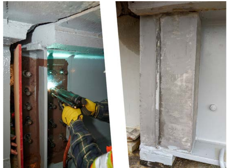
Repair of a deteriorated steel bridge beam end using UHPC. Source: University of Connecticut
