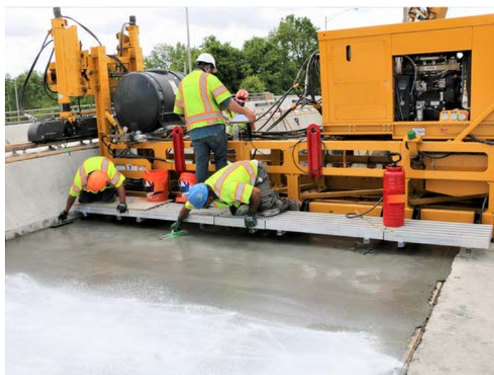
Installation of a UHPC overlay.
