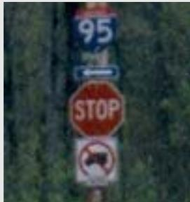
Answers: These signs are not mounted on the correct fixtures or mounted independently of each other. See 2A.16, 2A.18, and 2B.06 of the MUTCD.
