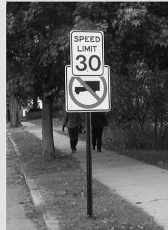
Section 2A.16 of the MUTCD states that “Signs should be individually installed on separate posts or mountings except where (a) one sign supplements another, (b) route or directional signs are grouped to clarify information to motorists, or (c) regulatory signs that do not conflict with each other are grouped, such as turn prohibition signs posted with one-way signs, street name signs posted with a stop or yield sign, or a parking regulation sign posted with a speed limit sign.”
