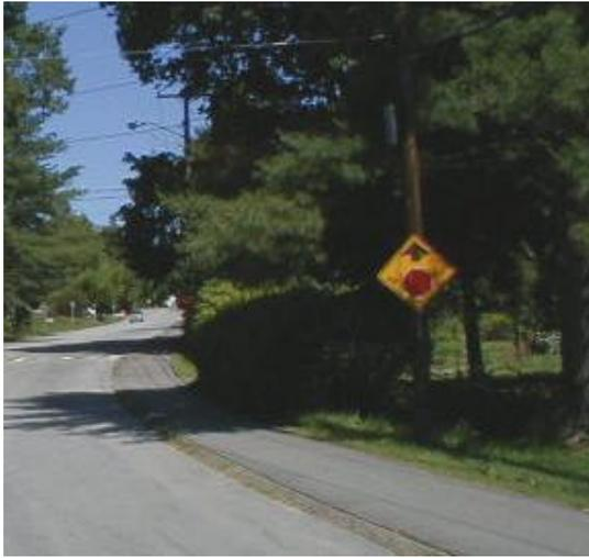
Figure 2. A properly installed Stop Ahead (W3-1a) sign.
