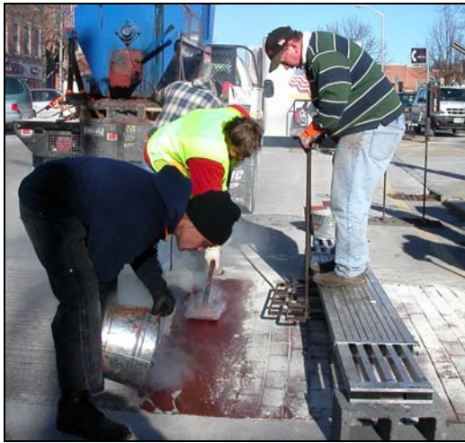
New crosswalk installation in Dover.
