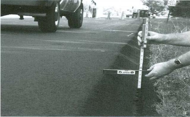
*Solution to drop-off from reconstruction or resurfacing projects: Install a 30- to 35-degree safety edge (wedge) during resurfacing, as in photo (courtesy of FHWA).*
