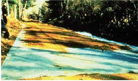
*Geotextiles help to stabilize roads with inadequate road bases*
