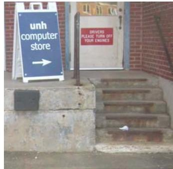
*Left: An inaccessible entrance to a public building. When rehabilitating this building compliance is necessary.*
