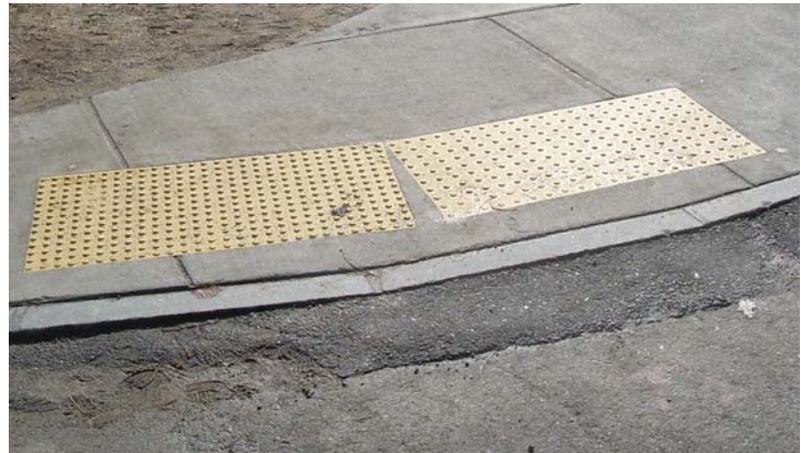
*These truncated domes aren't set correctly, they must span the curb cut width.*
