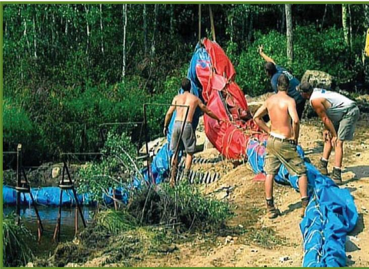
The town of Hollis used a portadam during a bridge replacement to provide temporary and semi-permanent barriers for water retention. Jeffrey Babel, public works director, Hollis, recommends the temporary daming system. Temporary dams are made of synthetic fabric and are low impact, which allowed the Hollis to use an expedited DES wetlands permit.
