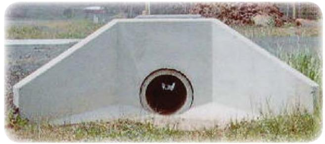
Figure 5: Header with Wing Walls
