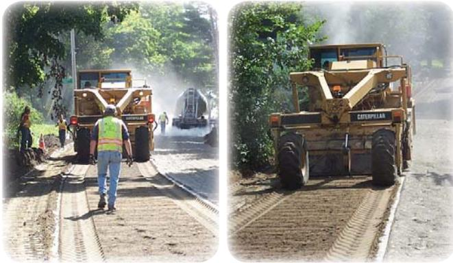
Eleven hundred feet of Norway Hill Road in Hancock underwent full-depth reclamation (FDR) this summer. FDR is the recycling of old road material by crushing and mixing it with cement and water then compacting it to create the base for a new road.
