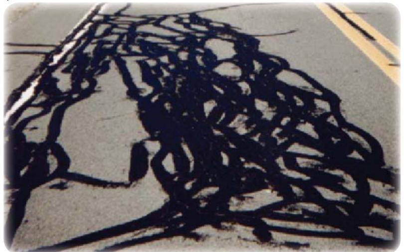
Figure 1: Crack sealing performed on alligator cracking. An alternate solution should have been used on this road.
