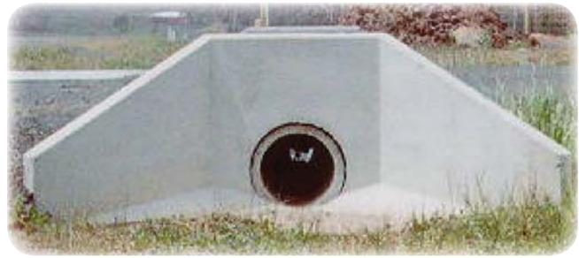
Figure 5: Header with Wing Walls
