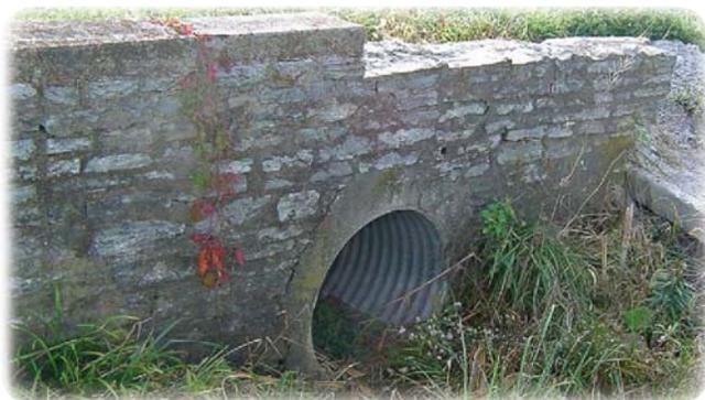
Figure 4: Typical Headwall
