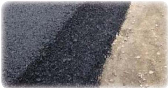
*Illustrating the taper between the roadway pavement and graded shoulder. Photo courtesy of Gary Antonelli, President, Advant-Edge Paving.*
