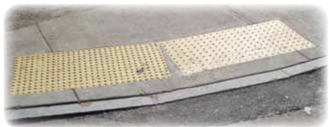
These truncated domes are not set correctly - they must span the curb cut width.
