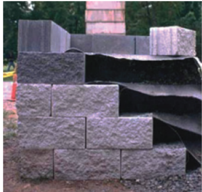
Typical geosynthetic reinforced soil system
