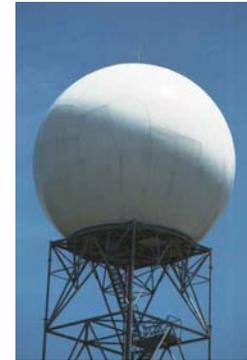
The radio waves reflected back to the antenna are converted to pictures to show the location and intensity of precipitation. To determine the direction of the precipitation and winds, the radar measures the frequency change in the returning radio waves. Waves of something moving away have a lower frequency while those approaching a radar will have a higher frequency.
